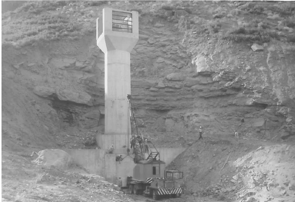
Figure 3.—Original construction photograph of the outlet works intake structure.
