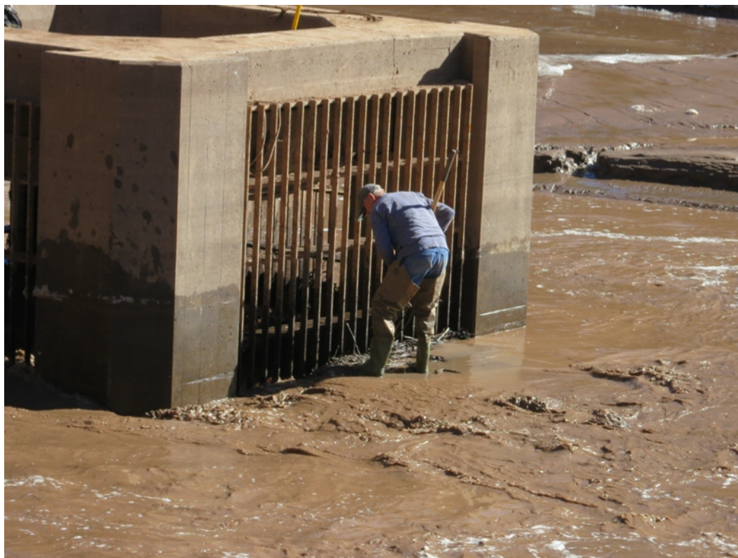
Figure 10.— Clearing sediment and woody debris from the intake structure in 2014.
