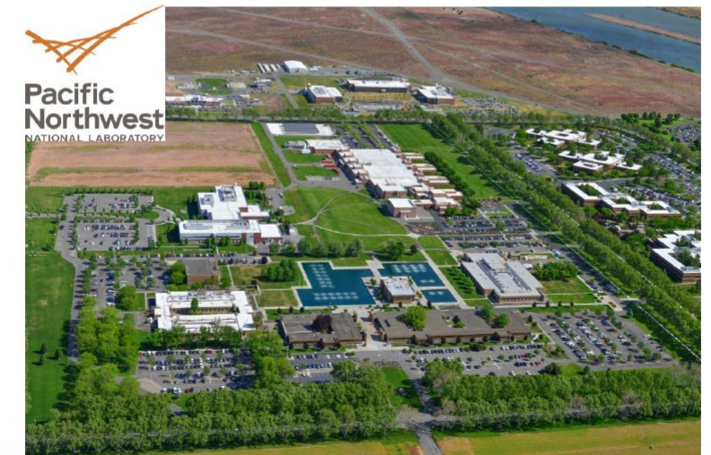
Figure 1: PNNL main campus, looking north.
