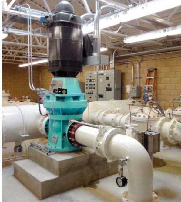
Figure 4. In-conduit hydropower turbine installed in a California water distribution system conduit
