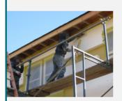
Applying Exterior Insulated Finish Systems (EIFS) is a multi-step, temperature reliant, one-off, labor intensive process using cost-burdened products.
