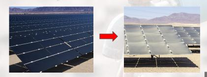
Due to soiling, solar plants can suffer about 80% loss in energy yield unless they are cleaned frequently.
