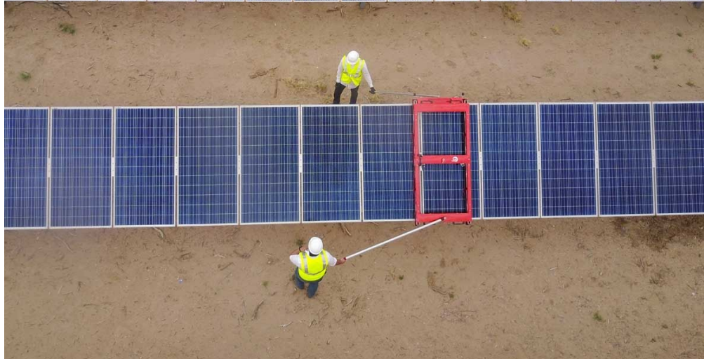
Figure 2. Two technicians pushing the MiniMax across an array of solar panels
