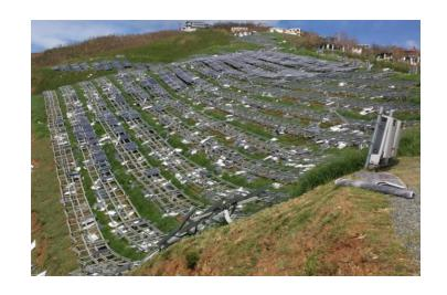
Solar panels are in harms way during hurricanes. Why is there not a procedure for removal to protect the most valuable asset? The ability to regain or maintain power after a hurricane is critical for recovery.
