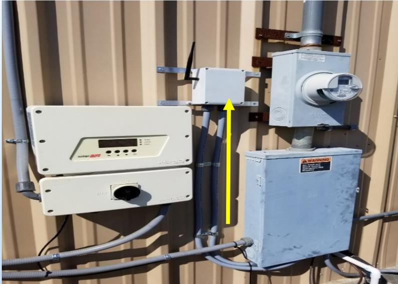
Apolloware CD – Delivers near real time revenue accuracy data on electric, gross and net solar generation via power line, Ethernet over customer IP or cell
